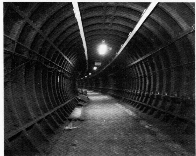
The old northbound City Line. Photo Nick Catford
